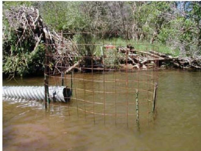
5. **Horizontal Cylindrical Wire Mesh Beaver Guard:** This alternative is used for various sized culverts. There is a large amount of surface area with allows more time between cleanings. It is the simplest design, easily constructible, and low cost.
